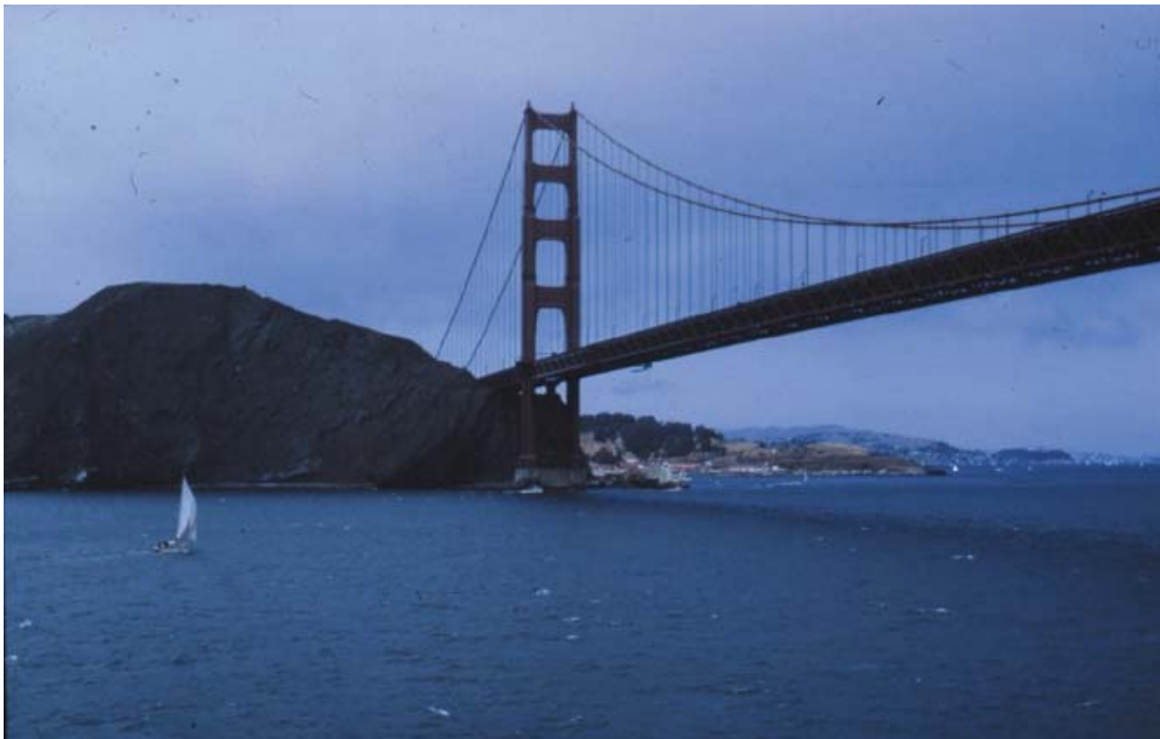
Golden Gate Bridge
